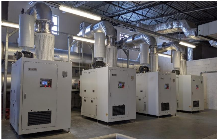
Figure 2-22 – High Speed Turbo Blowers
