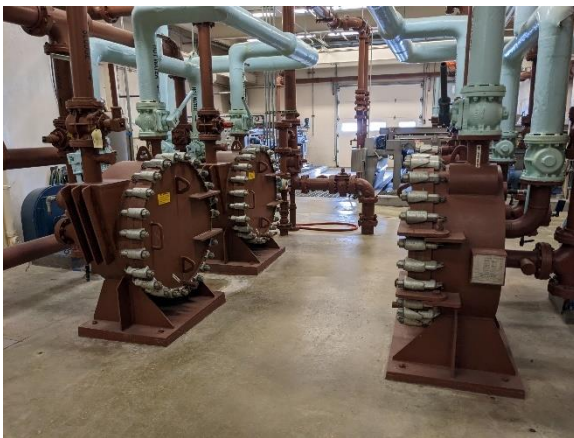
Figure 2-31 – Heat Exchangers
