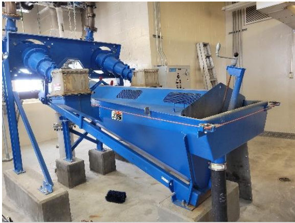
Figure 2-25 – Hydro-Cyclone Grit System
