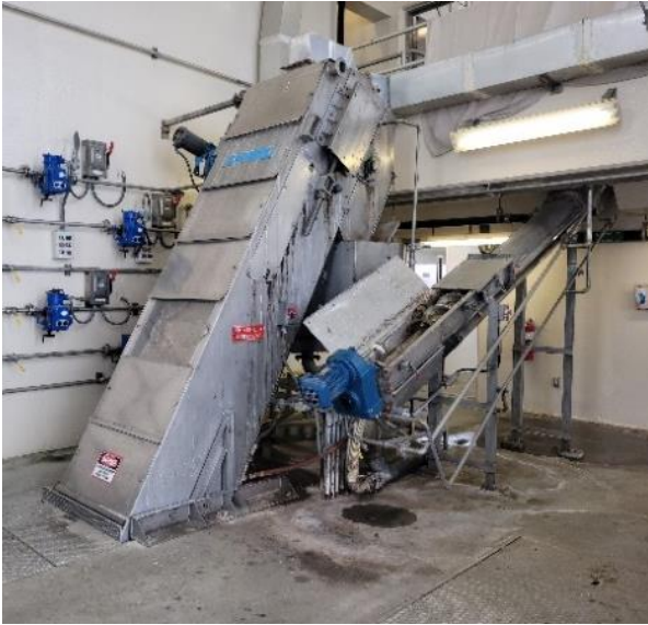
Figure 2-6 – Headworks Screen and Classifier
