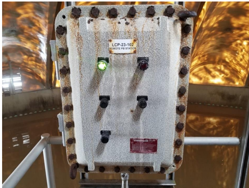
Figure 2-37 – Corrosion within Fermenter
