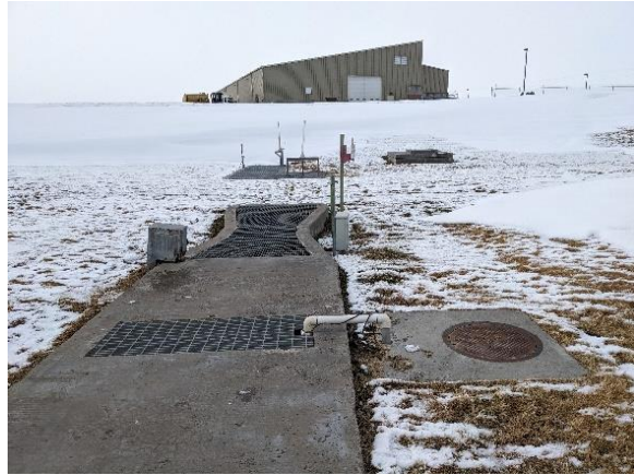
Figure 2-21 – Parshall Flume and Bisulfite Dosing
