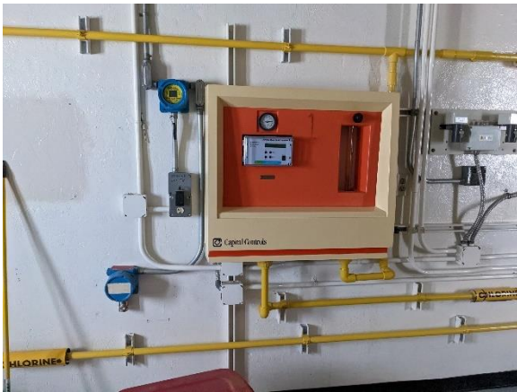
Figure 2-18 – Chlorinator #1
