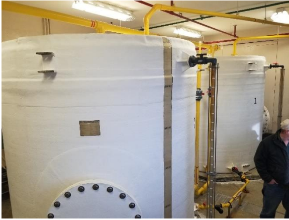
Figure 2-20 – Sodium Bisulfite Tanks
