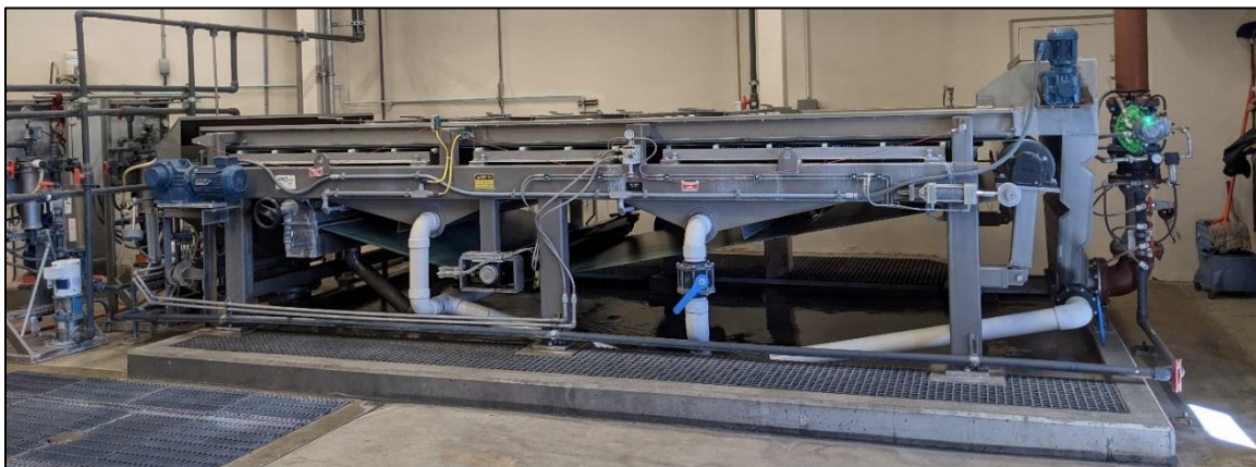
Figure 2-38 – Gravity Belt Thickener
