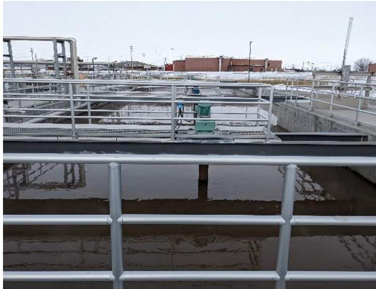
Figure 2-12 – Anaerobic Selector Basins
