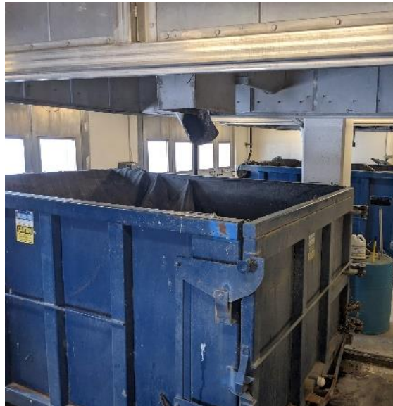
Figure 2-8 – Screening and Grit Dumpsters
