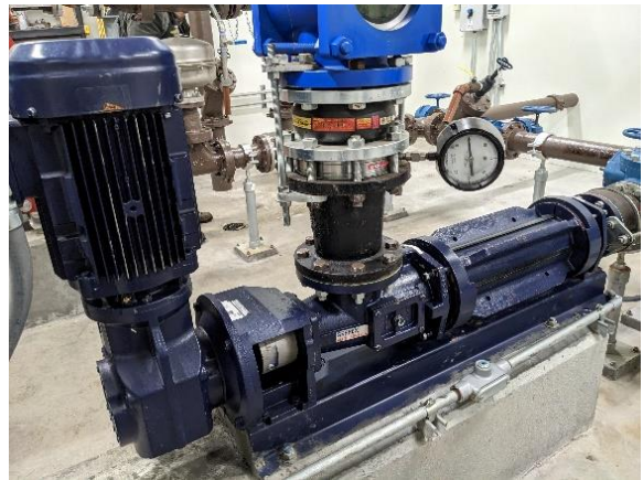
Figure 2-26 – Thickened Primary Sludge Pump
