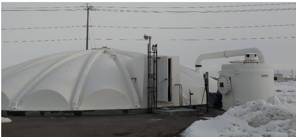
Figure 2-27 – Primary Solids Thickener/Fermenter
