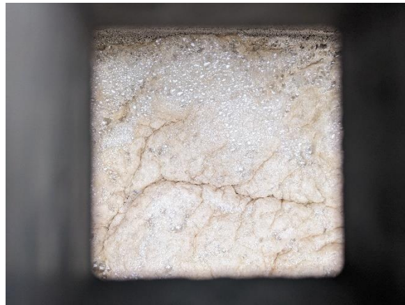
Figure 2-19 – Chlorine Injection Point Foam
