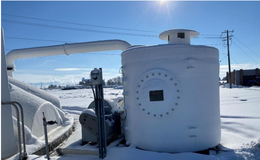
Figure 2-36 – Odor Control System
