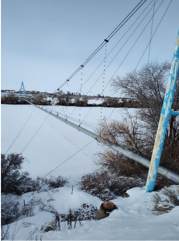
Figure 2-1 – Suspended Influent Line
