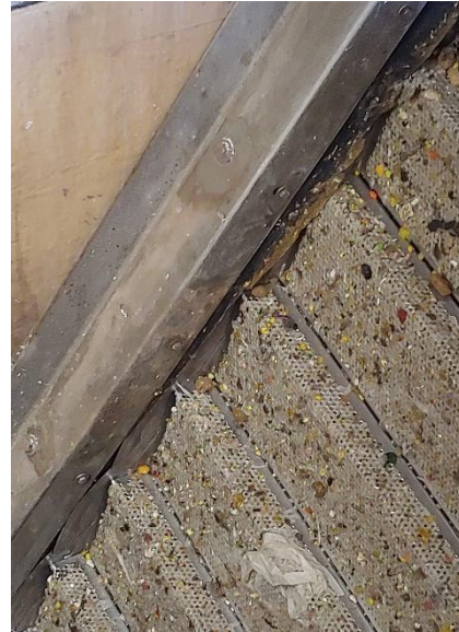
Figure 2-7 – Screen Side Seal
