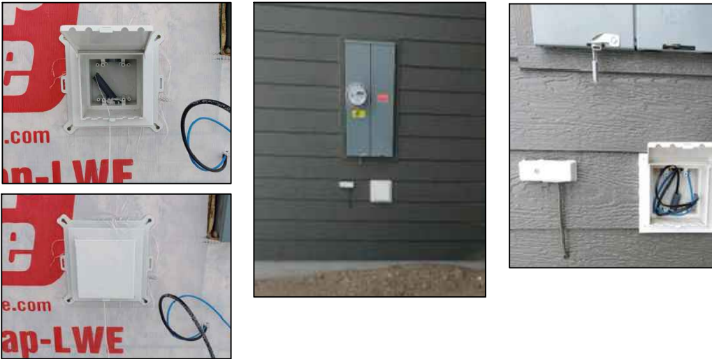
EXAMPLE 3 OF EXTERIOR COMMUNICATION WALL MOUNT
