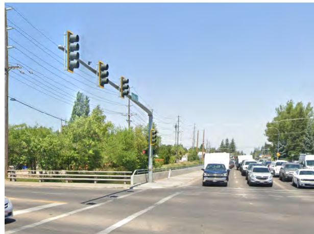
Figure 40 - Signal Mast Arm with No Overhead Lighting
