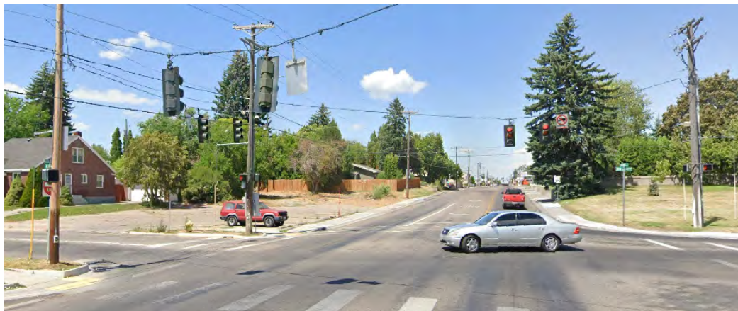
Figure 46 - Span Wire Signal at John Adams Parkway
