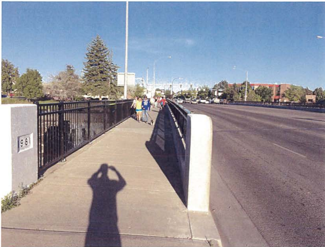
Path railing (river side) and traffic barrier concept at the Broadway Bridge (proposed to be installed at Pancheri)
